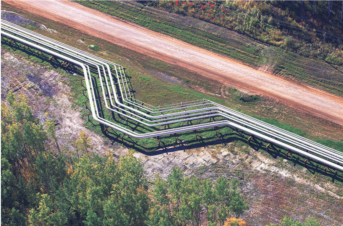
Suncor is working to reduce the cost, energy demands, and scale of critical equipment such as the steam generators (top) to allow future expansions, increasing the flow through its pipelines (lower). Source: Suncor.
